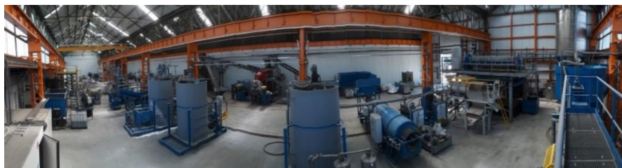
Figure 1: General view of the SOLINDUS platform
