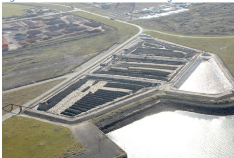
Figure 2. Pretreatment of the sediments: dewatering of sediments by lagooning (left), on site pre-treatment of lagooned sediments with a CSA additive.
