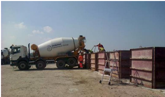
Figure 3. Pouring of the concrete blocks
