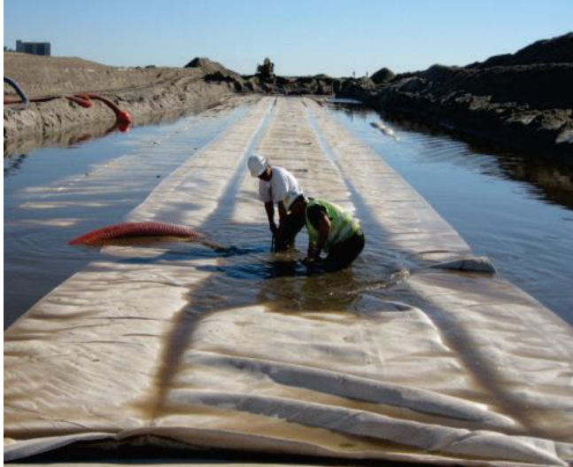
Figure 1. Filling of geotubes with sand, underlying the western breach.
