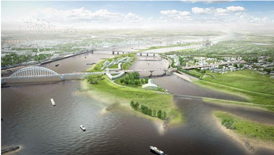
Figure 1 Room for the River
