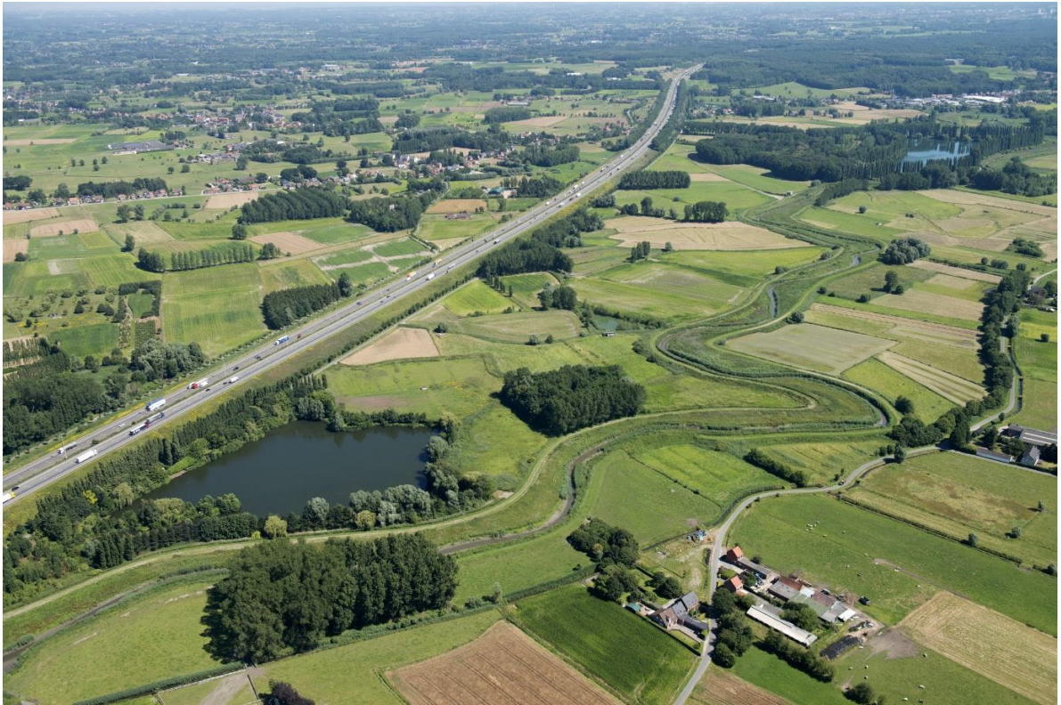
Figure 1. Project area seen from the south
