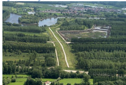
Figure 4. Finished Compartment dyke
