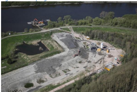
Figure 3. Site view during works
