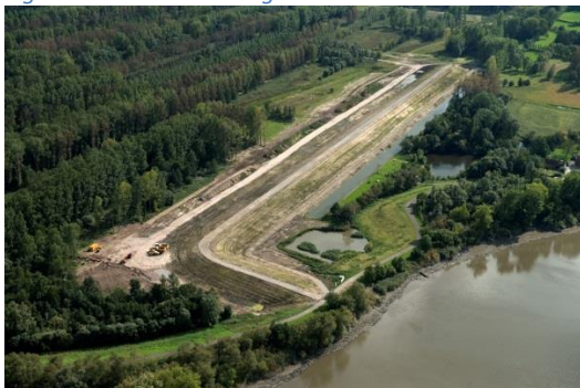
Figure 5. Finished Primary dyke
