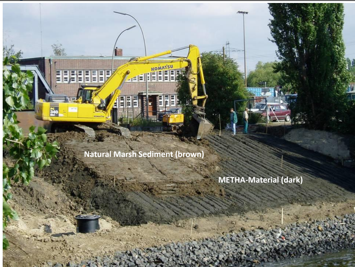
Figure 1. Photo of pilot dike construction using METHA Material below a layer of natural marsh sediment in 2004. Photo by J.Gebert.
