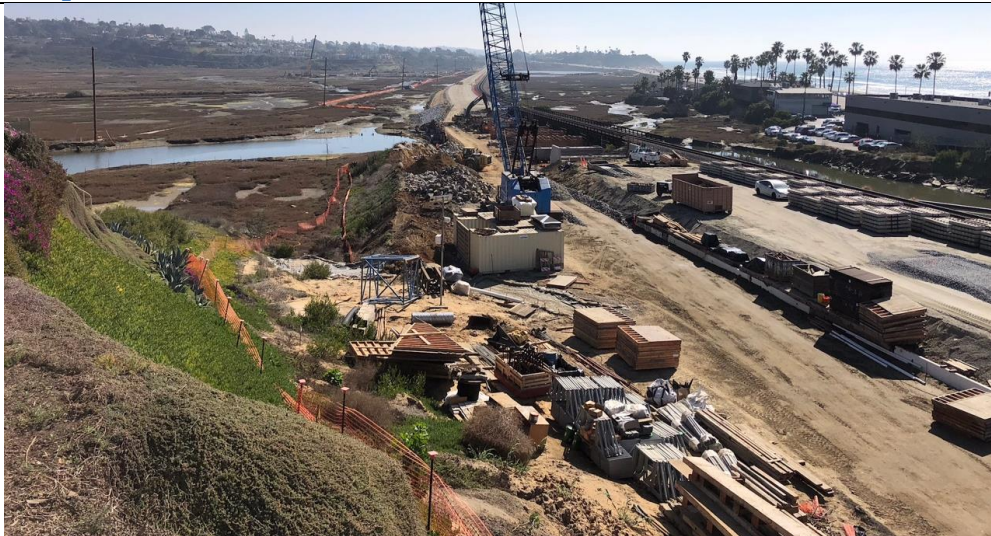
Figure 1. Rail Corridor Construction (foreground), with Containment Pit in Preparation ( background)
