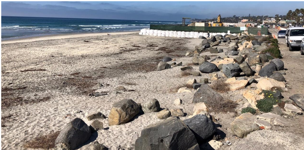
Figure 3. Sediment Stockpiling and Staging Area, San Elijo State Beach
