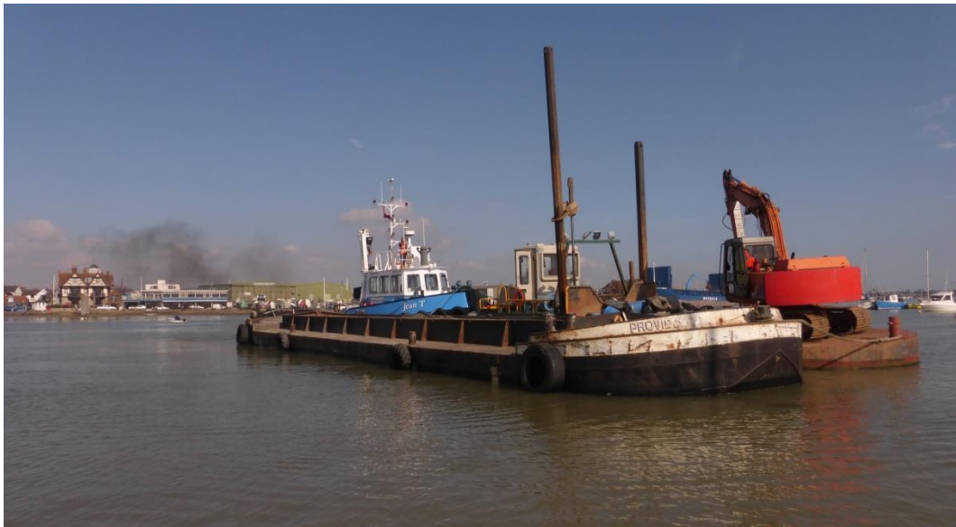
Figure 2. Mechanical dredging and hopper barge transport to the restoration compartments (Figure 1).
