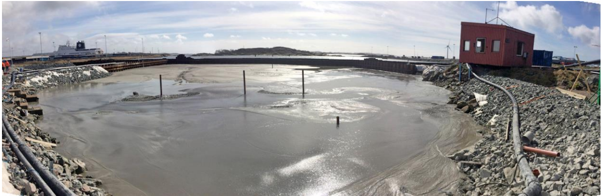
Figure 1. Sediment stabilised with GGBS:cement binder in Gothenburg Port Arendal Field Trial
