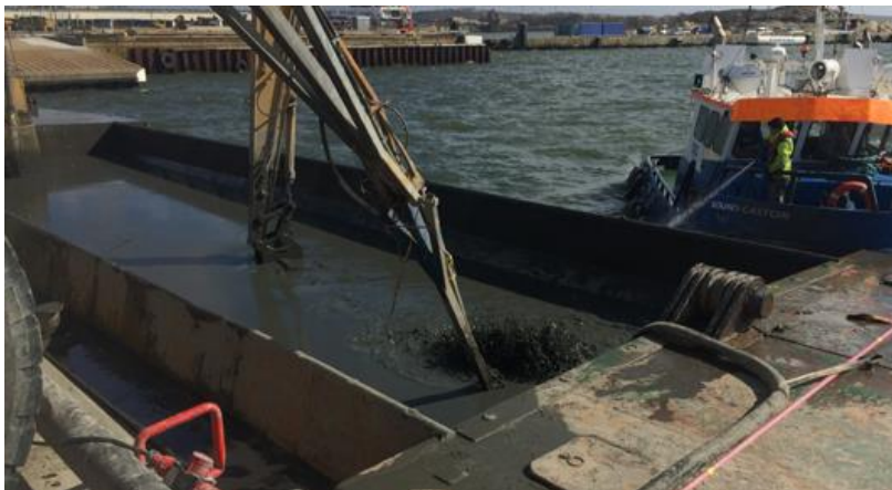
Figure 3. Sediment being homogenised in barge prior to mixing with binder
