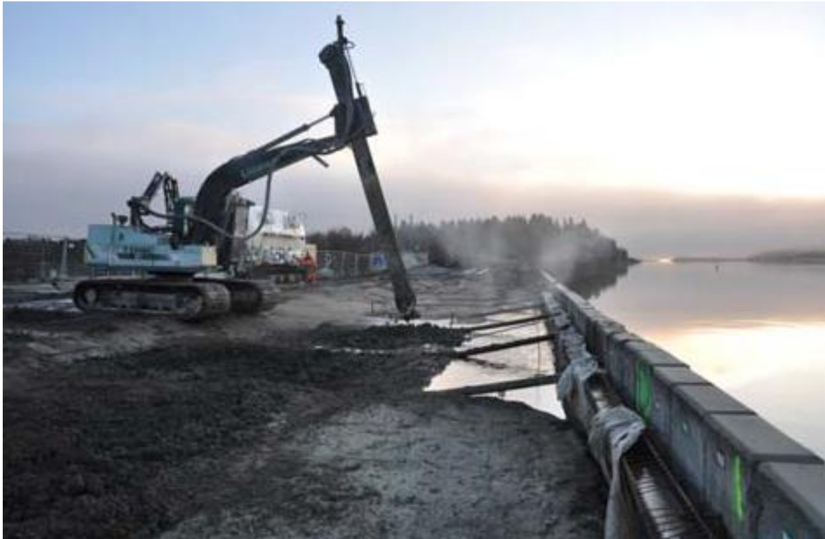
Figure 1. Mass stabilisation of dredged contaminated sediment behind concrete quay wall
