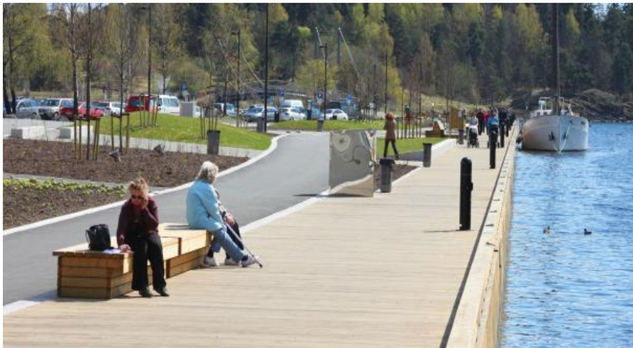
Figure 2. Completed project – stabilized sediments form new quay wall and walkway
