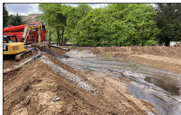
Figure 3. Discharge into the upper lagoon. May 2021.
