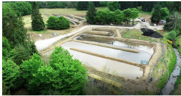
Figure 1. Aerial view of the lower lagoon, with the upper lagoon visible in the background. June 2021.
