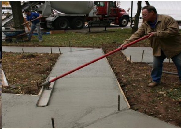
Figure 4: Poured concrete sidewalk
