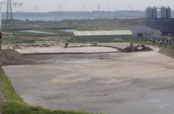
Figure 4: removing clean sand from the basin
