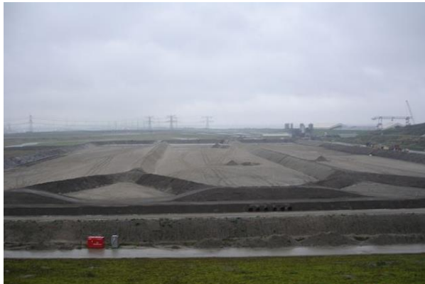
Figure 1: Construction of the sand separation basins (2006)
