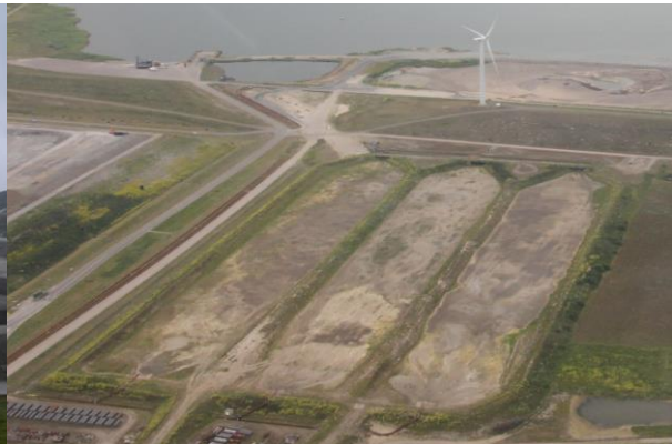
Figure 2: Aerial view of the basins (2017)
