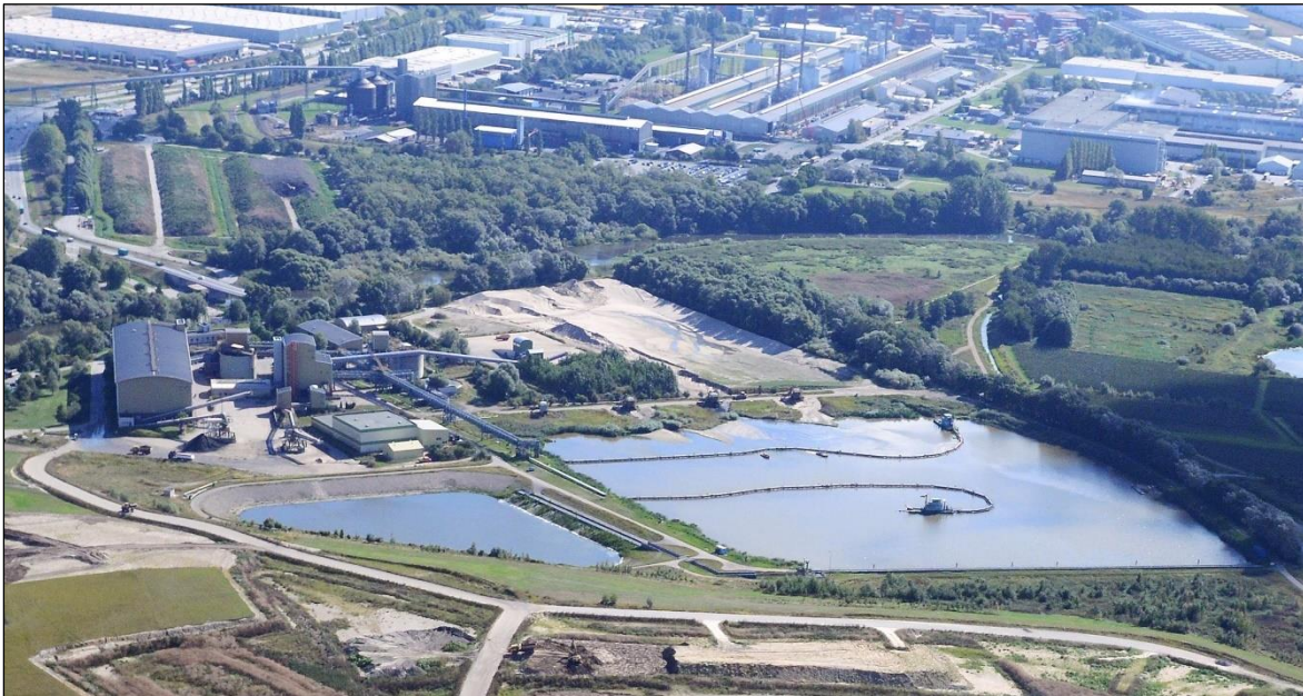
Figure 3: Aerial photograph of METHA-Plant Hamburg
