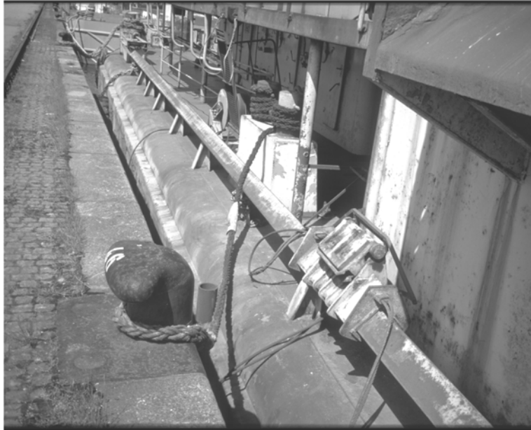
Figure 5-13 Sliding part of the Barge Hauling installation
