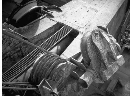
Figure 3. 77 Side wire sheaved in upwards position
