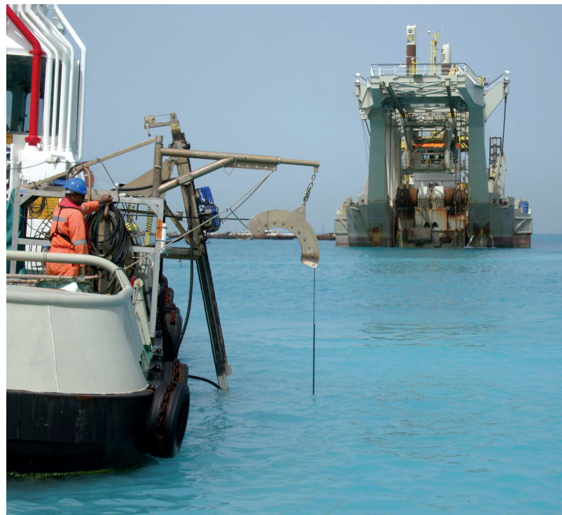
Figure 1: Monitoring during dredging
