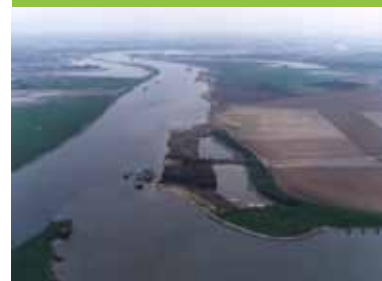
Dredging plays a role in enlarging the discharge capacity of rivers for flood management
