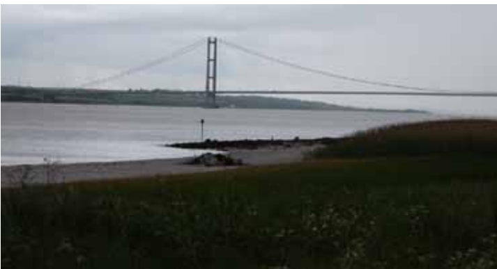
Measures to deal with expected sea level rise include managed retreat of sea defenses in the Humber estuary.
